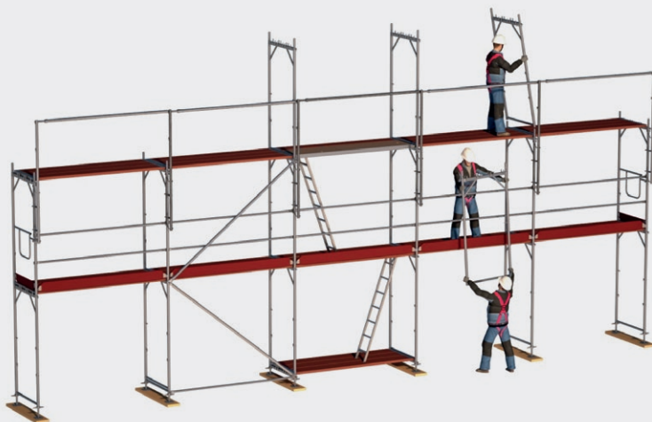
Figure 25: Example of vertical transport by hand
